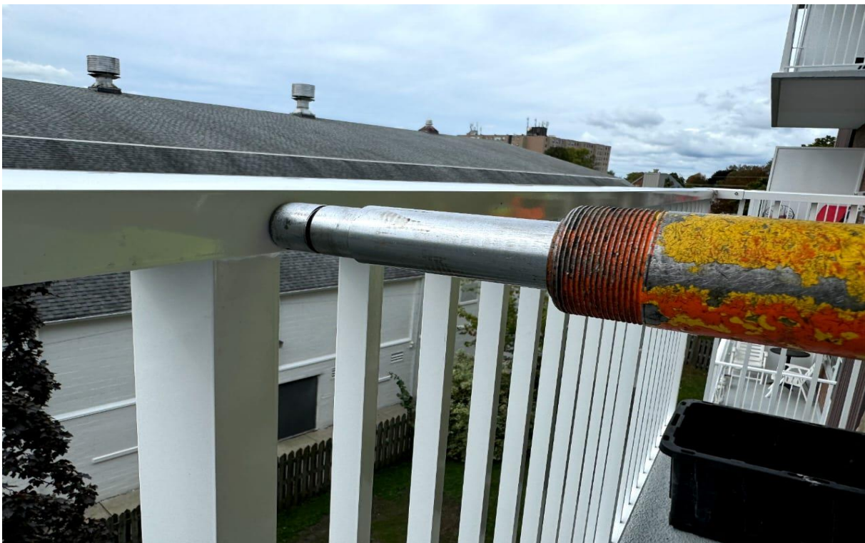
Photograph 4: Showing outward load application at the top of an intermediate post
