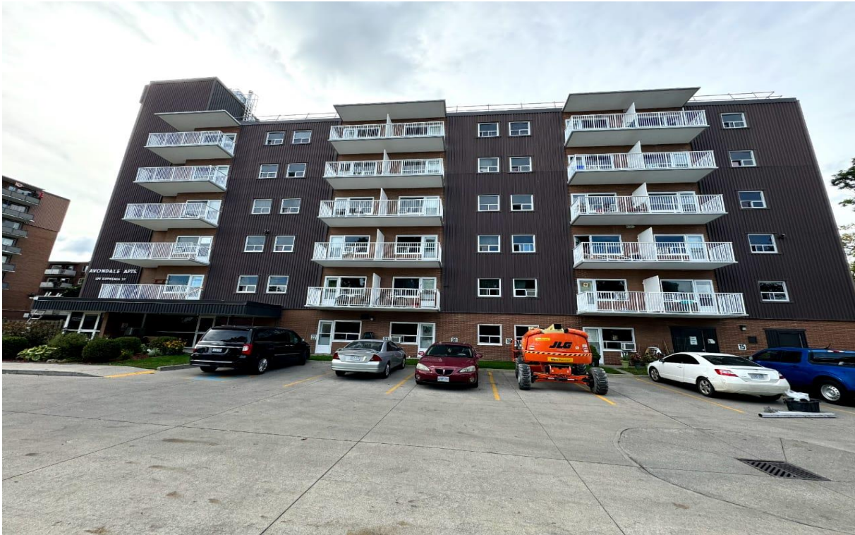
Photograph 1: General overview of the building
