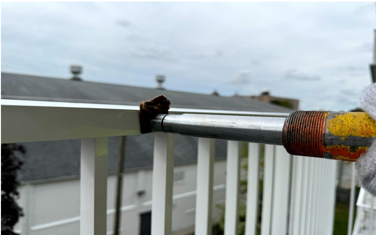
Photograph 8: Showing outward load application at the handrail mid-section
