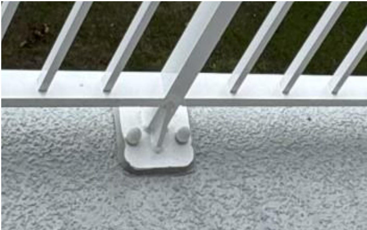
Photograph 3: Typical guardrail shoe detail
