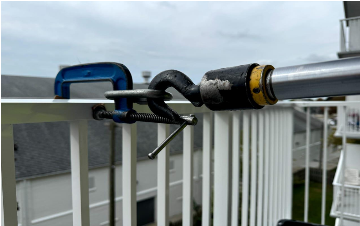
Photograph 9: Showing inward load application at the handrail mid-section
