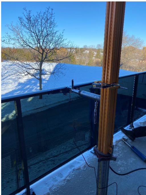
Photograph No. 7 Handrail Mid-section Outward Load
