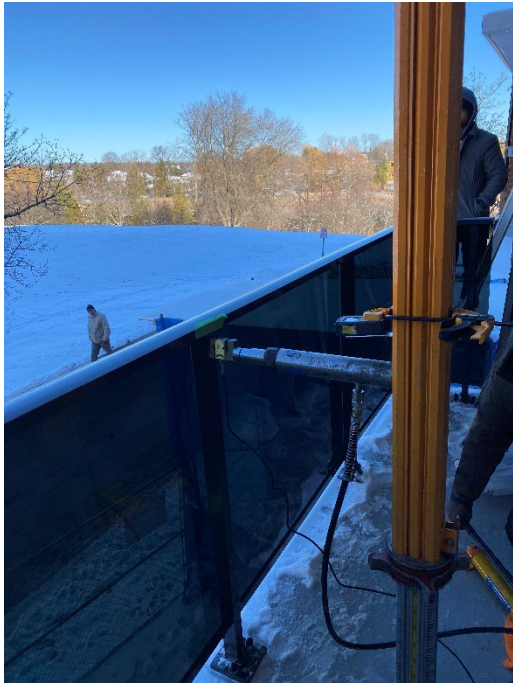
Photograph No. 3 Intermediate post Horizontal outward load (Top)
